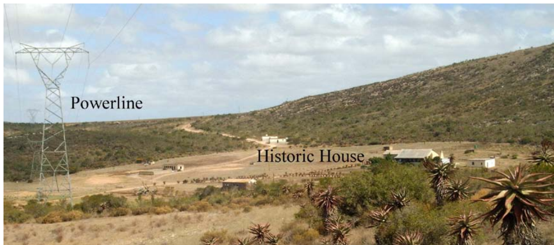
Figure 5. Position of existing 132kV powerline in relation to Diamant homestead
