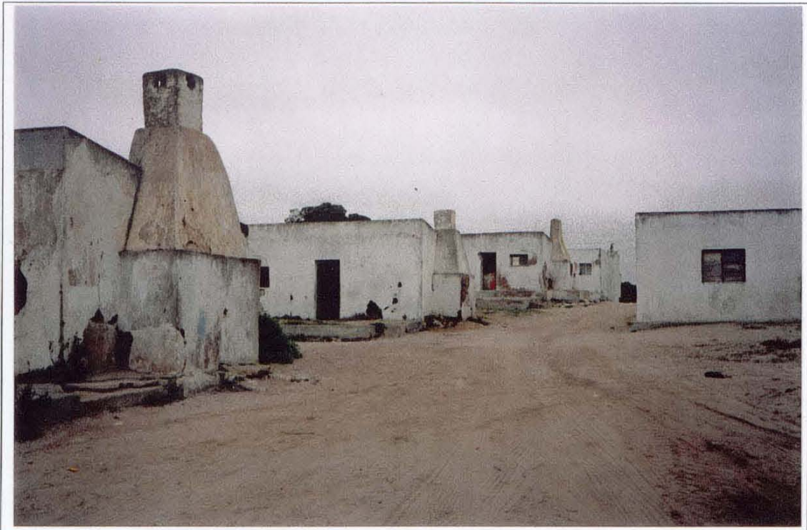
PLATE 3: One of the vernacular housing styles in the village with lean to roofs and end chimneys. These all seem to be constructed with a combination of brick types but some stone is also present.
