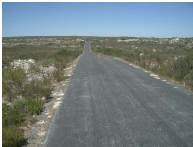
Figure 18. View of the powerline route facing north, taken from the Park Gate.
