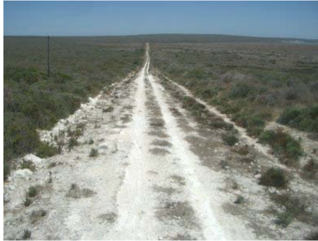
Figure 7. View of the route facing north west
