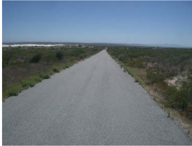
Figure 19. View of the powerline route facing north, taken from the Park Gate.
