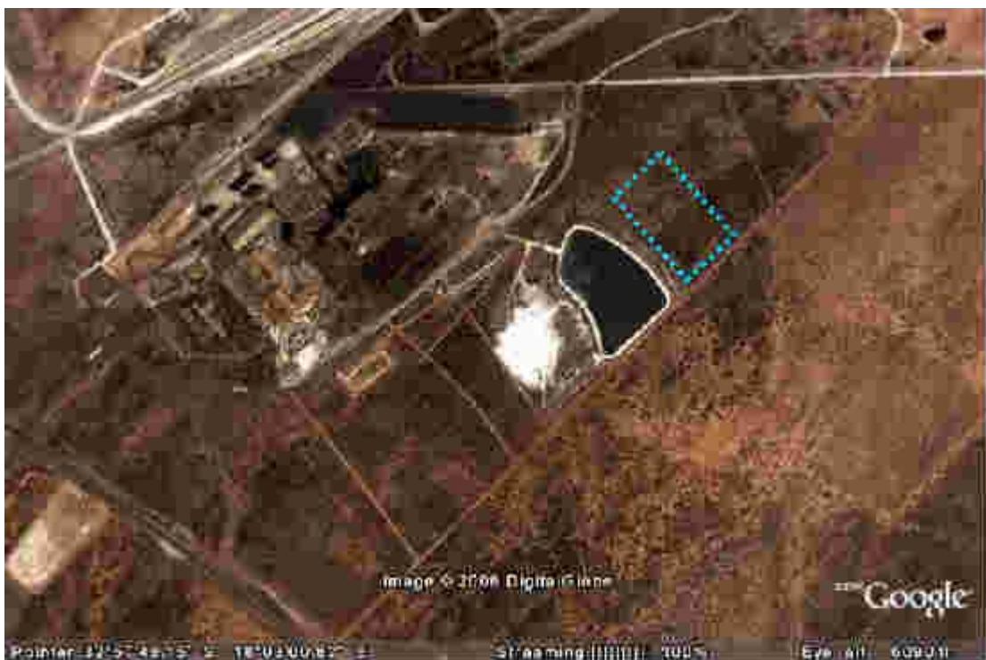
Site of proposed disposal dam, Namakwa Sands Smelter, Saldanha.
