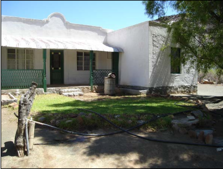
Fig.14 Farm house at Meintjieskloof is situated next to the road.
