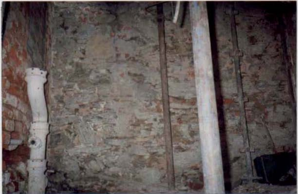
Plate 2: Some of the stone-walling revealed in the courtyard area during renovations.
