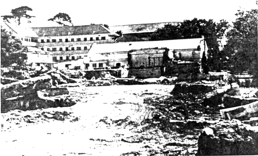
Photograph 1: Outline of the old mill core adjacent to the pumphouse
