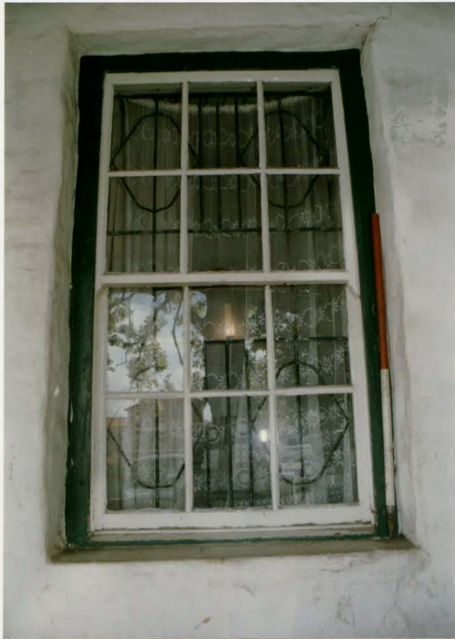
Figure 3.8: Sash window - detail.
