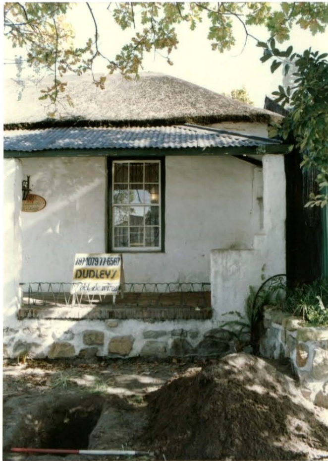
Figure 3.4: Front facade - detail.
