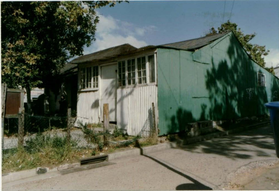
Figure 3.17: Corrugated iron structure.
