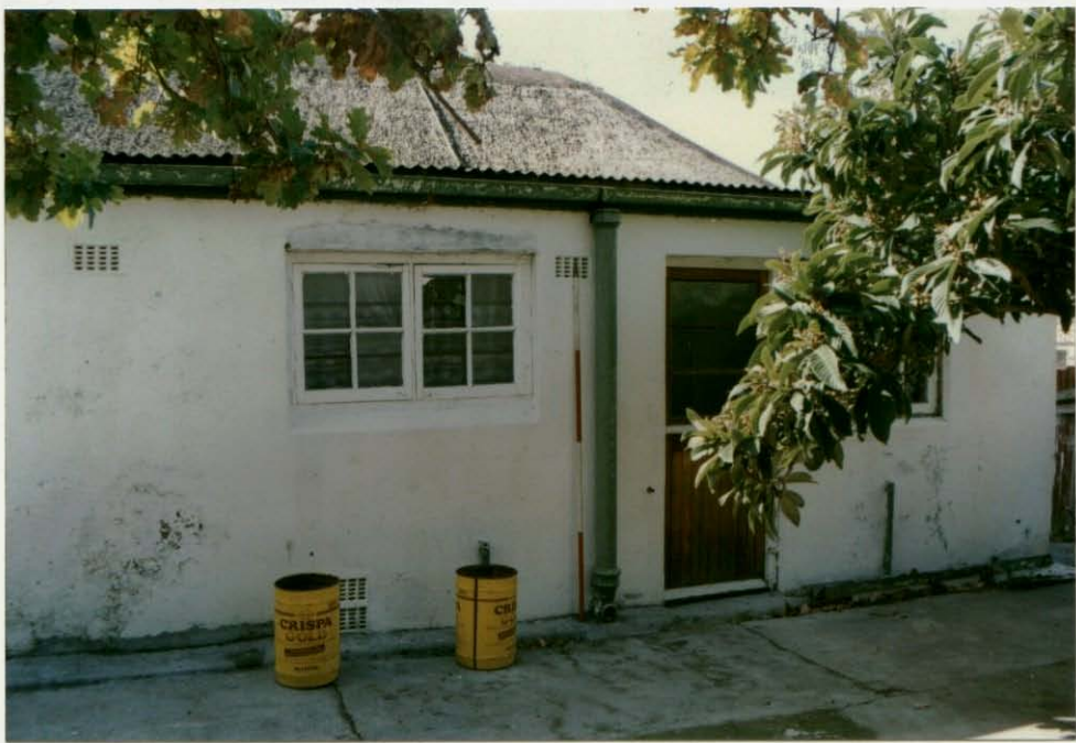
Figure 3.14: Rear facade - detail.
