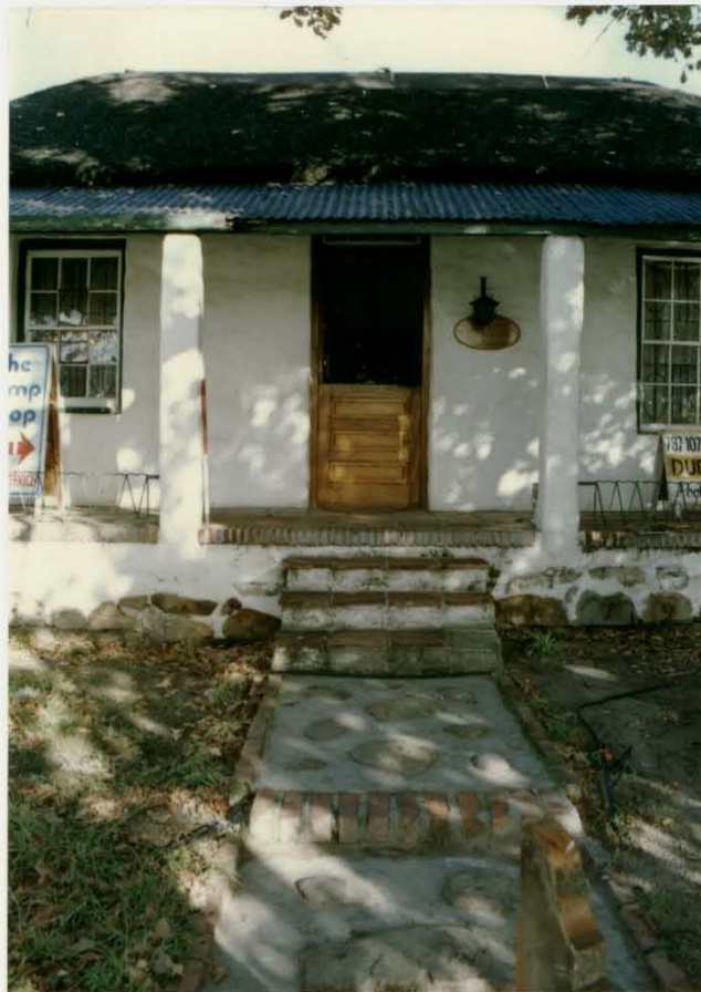
Figure 3.5: Front facade - detail.
