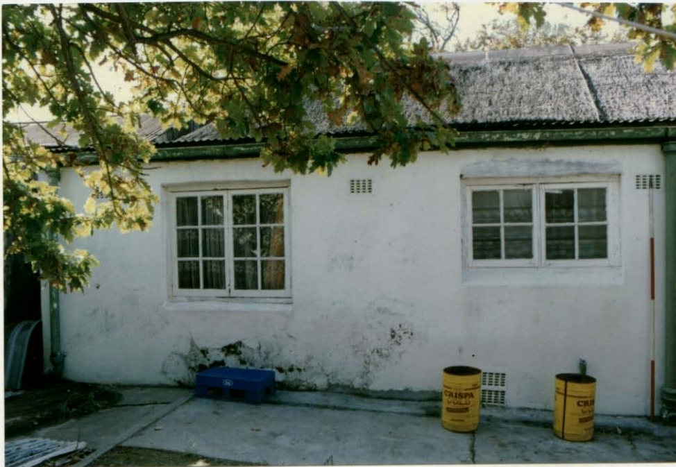
Figure 3.15: Rear facade - detail.
