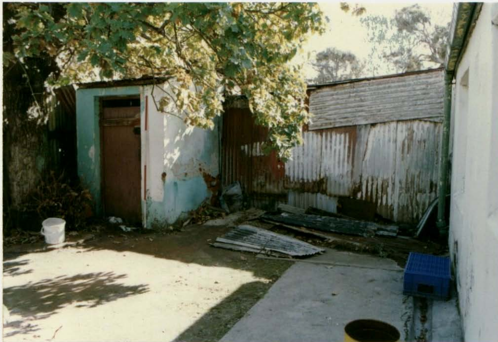
Figure 3.16: Rear yard with outhouse.
