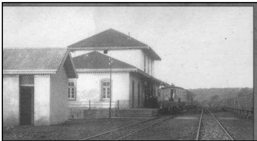
FIGURE 3: Ressano Garcia station in the early days. The main building, though changed, still exists.
