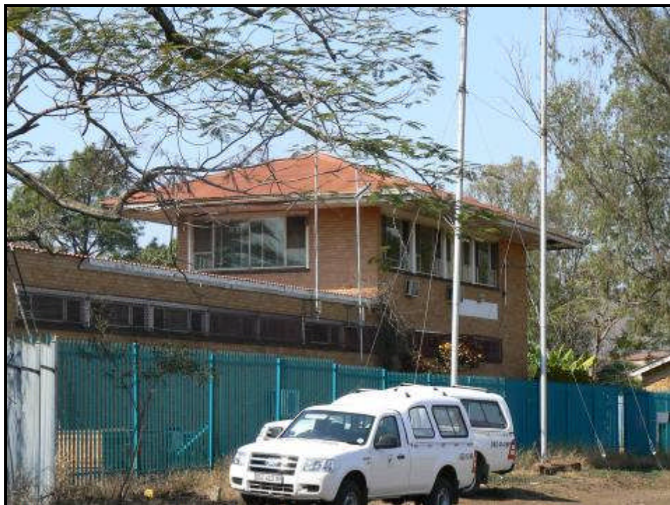
FIGURE 15: LB 6(2) Signal cabin (1960s) at Komatipoort Station
