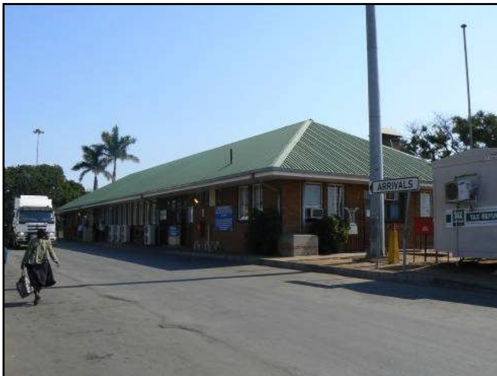
FIGURE 11: LB 3 Modern Lebombo border post offices
