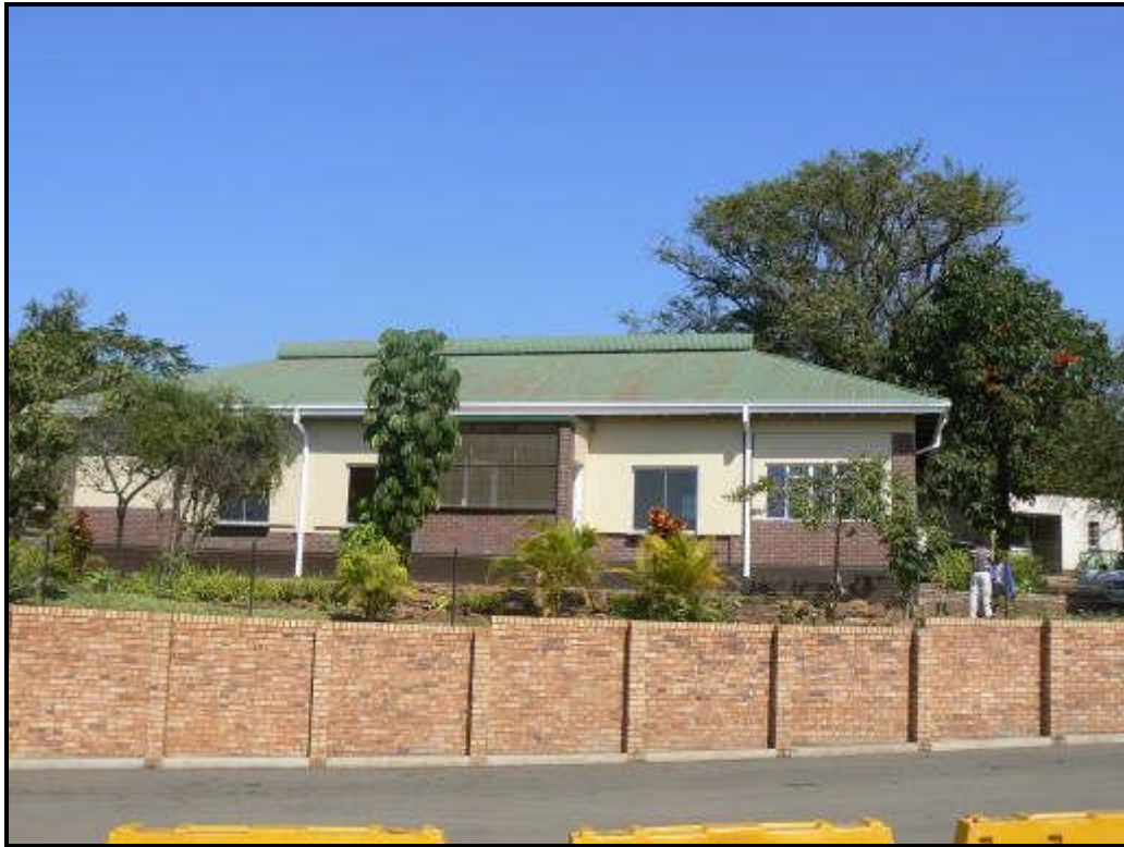
FIGURE 13: LB 5 Modern Lebombo border post staff quarters known as Buildings 116-156
