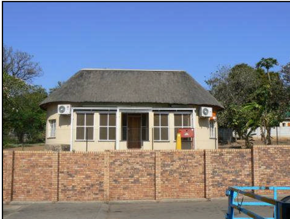
FIGURE 10: LB 2 Original rondavel-type staff houses (1930s), known as Buildings 114 and 115 at Lebombo Border Post
