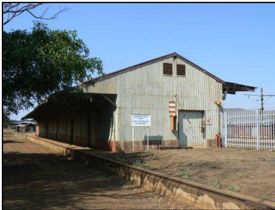
FIGURE 19: LB 6(6) Goods shed (early 20 th century) at Komatipoort Station
