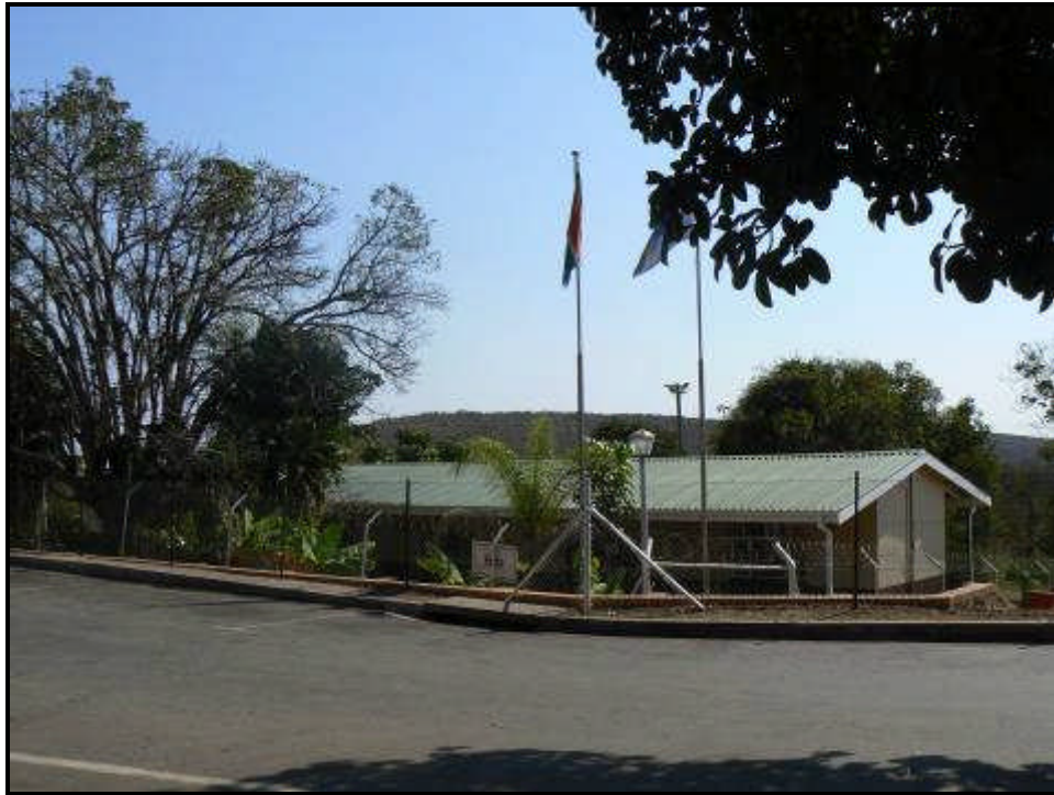
FIGURE 9: LB 1 modern buildings at Lebombo Border Post used by the SAPS and SARS
