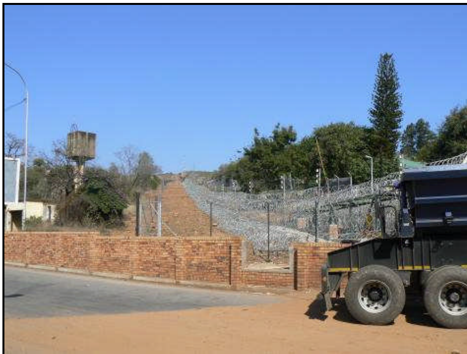
FIGURE 21: RG 2 Border fence, pumping station and water tower (extreme left) at Ressano Garcia
