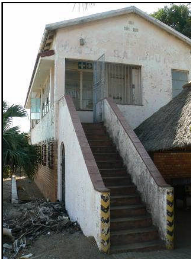
FIGURE 17: LB 6(4) Signal cabin (1950s) at Komatipoort Station
