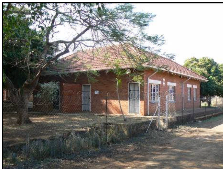
FIGURE 18: LB 6(5) 1940s building at Komatipoort Station
