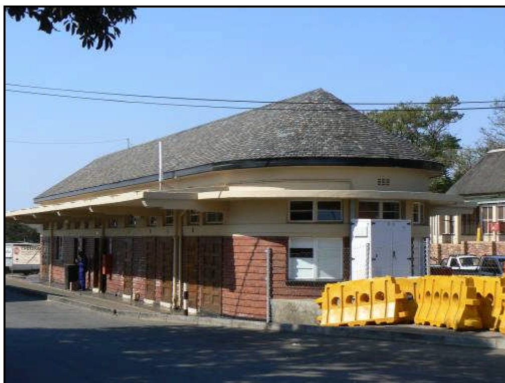
FIGURE 12: LB 4 Historic (1940s) Lebombo border post offices now used as toilets
