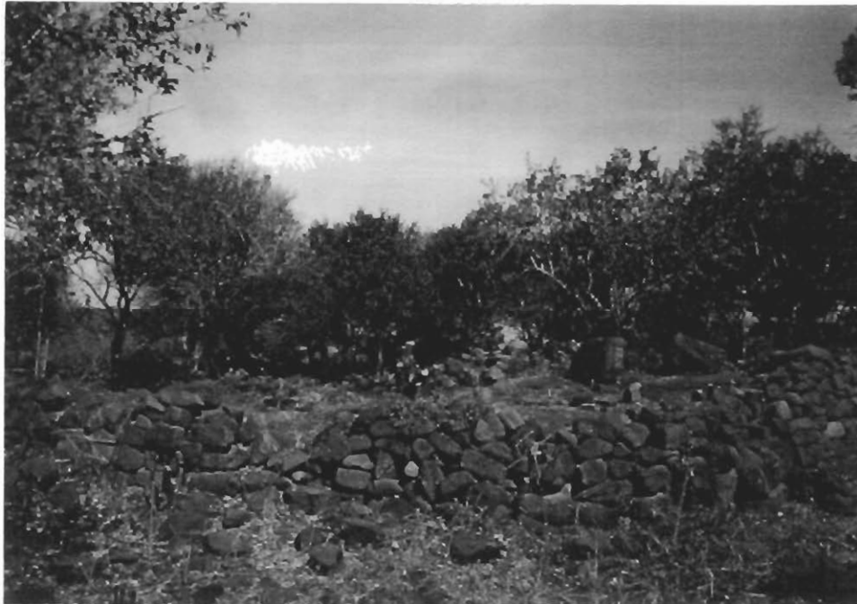
Figure 12. A view on the kgotla in Site SCH022.1. Note the large boulders used to built the entrance to this structure.
