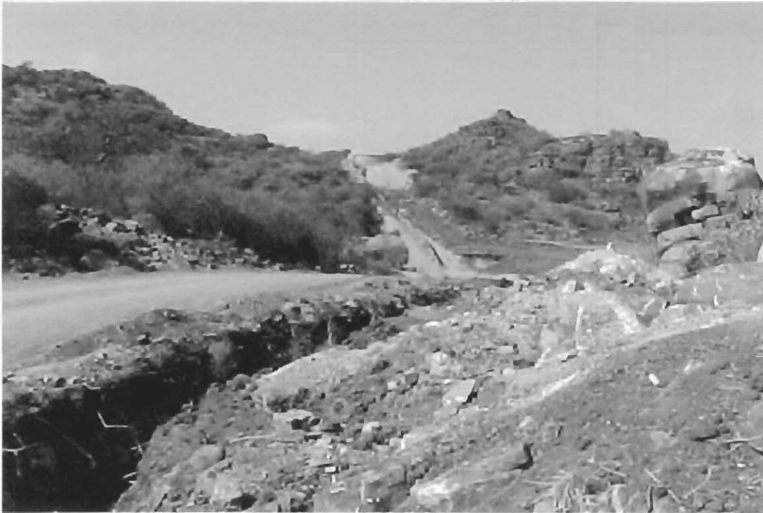
Photograph 1: The road and pipeline excavation through the Hoekfontein archaeological site.
