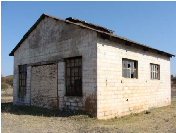
Figure 4 One of the old farm sheds at site no 1.
