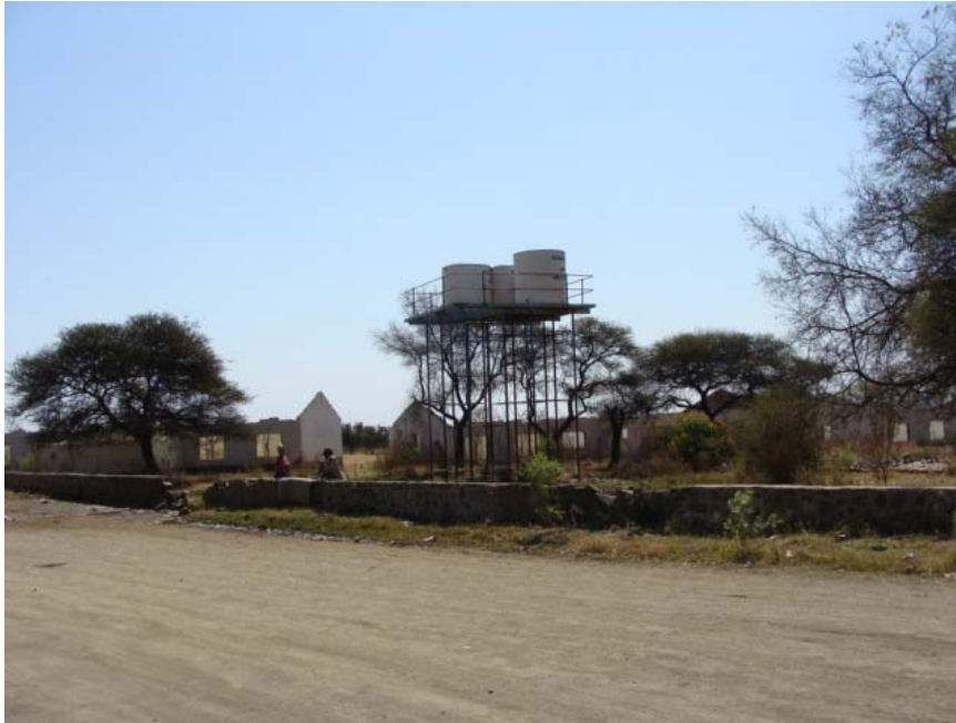
Figure 3 Old hostel on the eastern side of the surveyed area.
