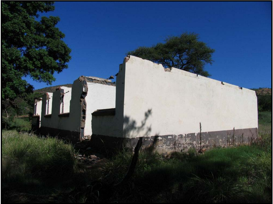
Fig. 4. One of a number of similar buildings on the site.
