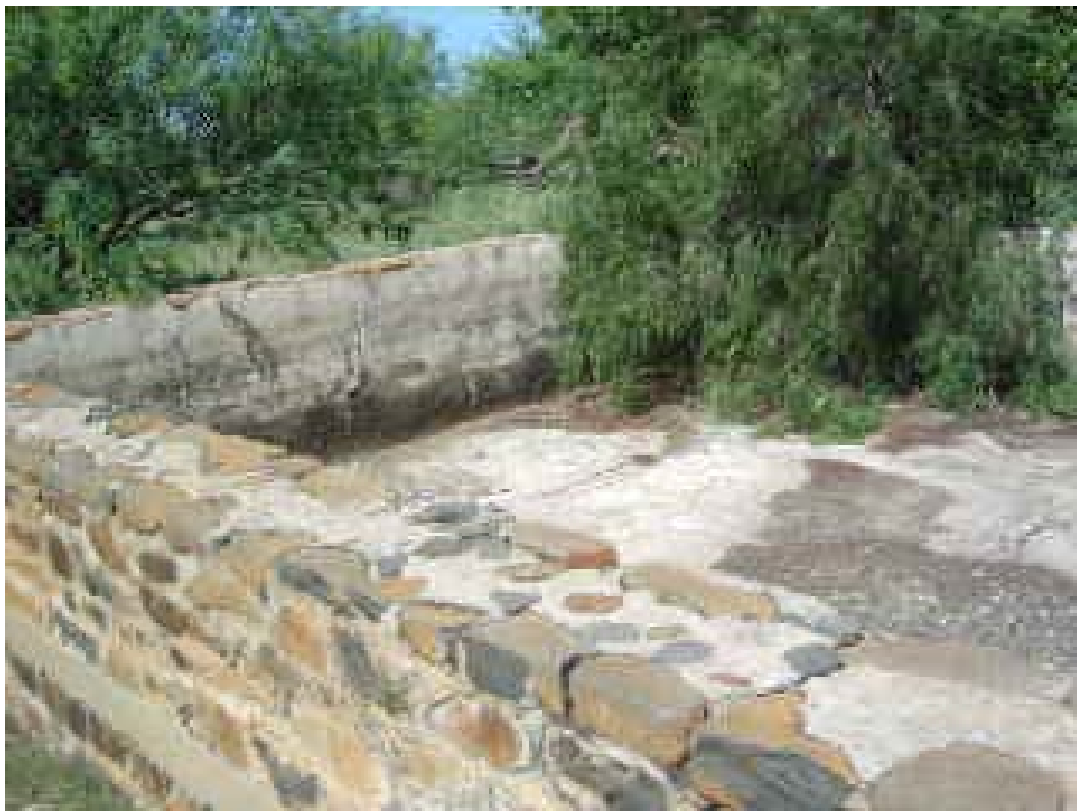
No 9. Remains of reservoir
