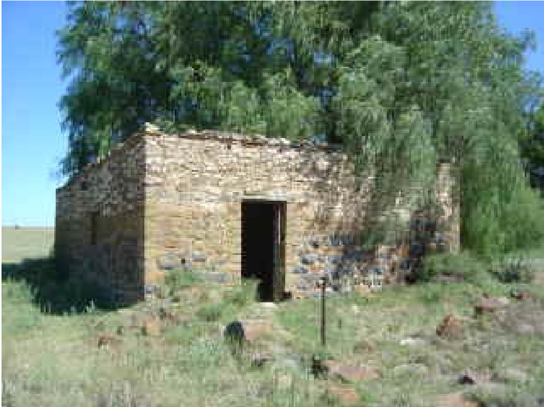
No 10. One of the outbuildings
