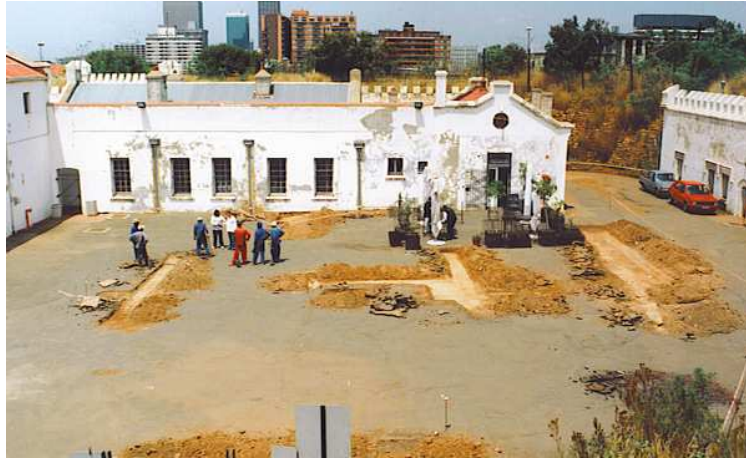
Figure 13. Excavation T04 and T05 in the central parade ground.
