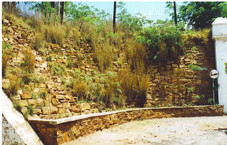
Figure 19. The south-western rampart today.
