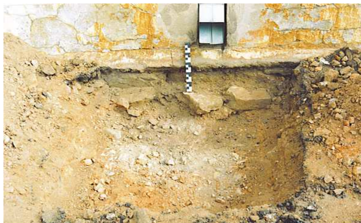
Figure 7. Rubble and building foundation visible in the extension of T01.
