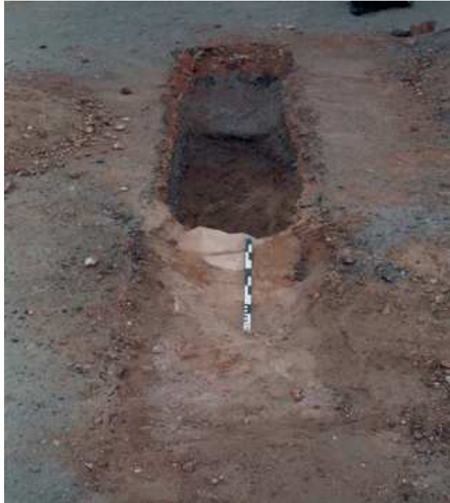
Figure 10. T03 with the stone foundation blocks in the foreground and the ashy landfill and water-pipe in the background.
