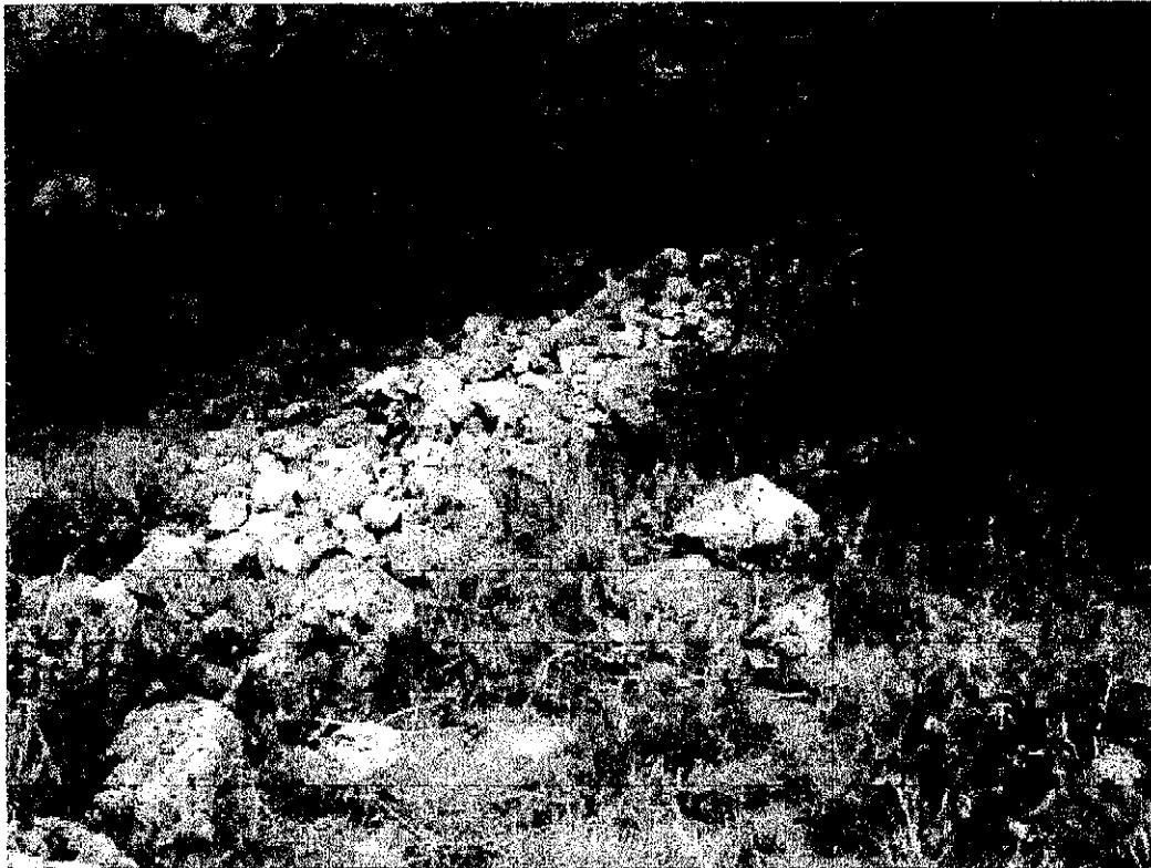
No. 1 Low stonewalling with rubble in the middle of the wall
