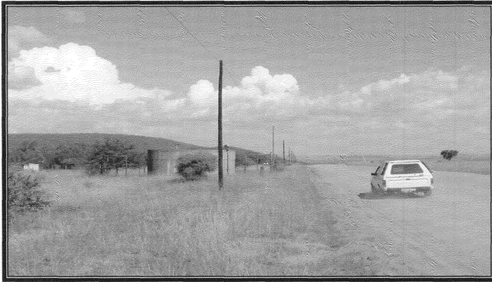
Plate 1: Makgadimeng water reservoir showing the road along which the pipeline would follow.
