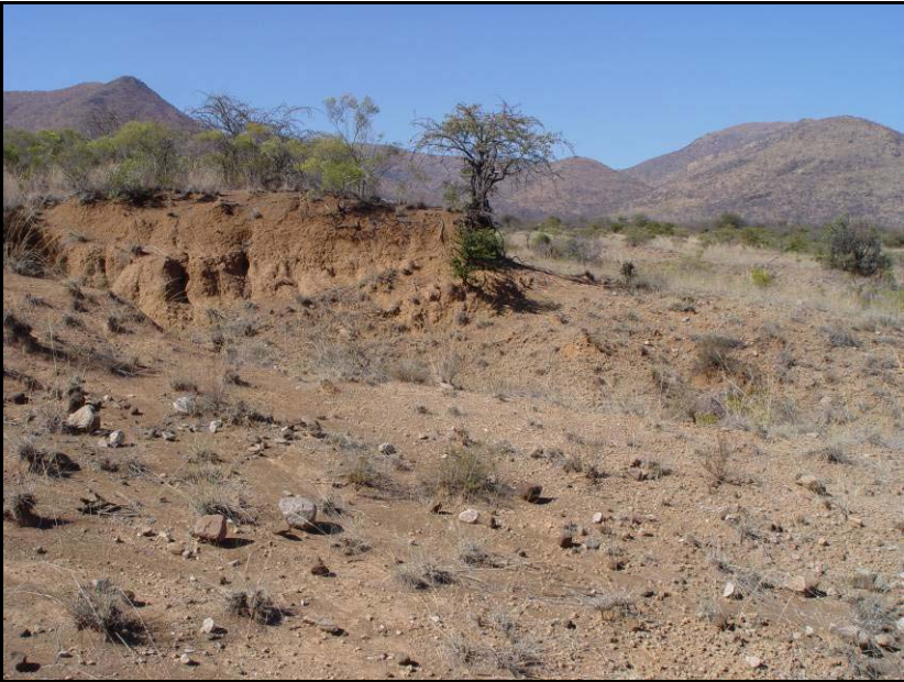
Figure 1: Surface erosion occurring in the area.
