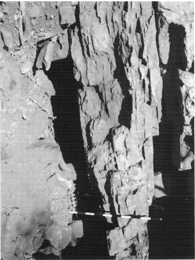
No. 4 Shaft entrance with two wooden poles supporting rock
