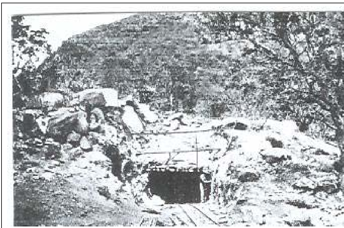
Figure 15- An incline shaft in operation on the Merensky Horizon during the early 20 th century (Wagner 1973:151) (above). The shafts on Onverwacht 292KT had similar appearances and were used to penetrate the Merensky Reef in order to obtain platinum bearing deposits from this horizon (above).
