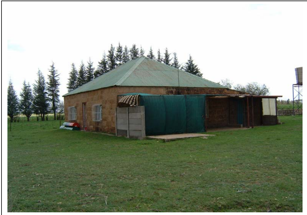
Figure 2- Historical House 01 (HH01) is located in the centre of MFC02 in the southern part of the study area. This house was built with sandstone blocks while the lean-to was also constructed with slabs of ferricrete.
