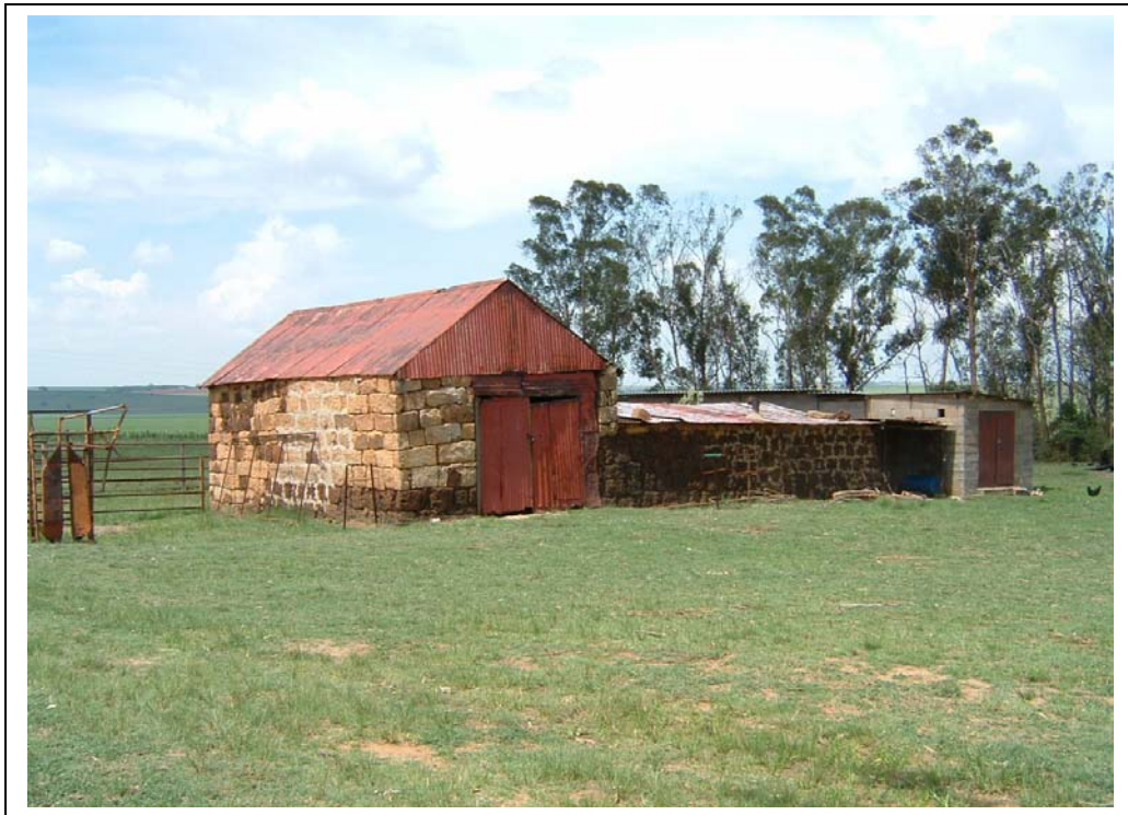
Figure 3- The outbuilding (shed) that is associated with Historical House 02 (HH02) is located slightly to the north of the historical farm homestead. Note the light-brown (sandstone) and dark-brown (ferricrete) blocks that were used to build the walls.
