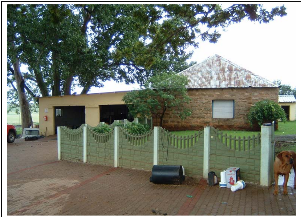
Figure 4- Historical House 02 (HH02) is located in the centre of MFC04. This house is situated next to a modern residence (not visible in the photograph) and is linked to a double garage (left).
