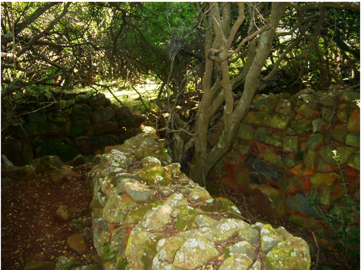
Fig. 4. Typical stone walling on a site similar to those under discussion.
