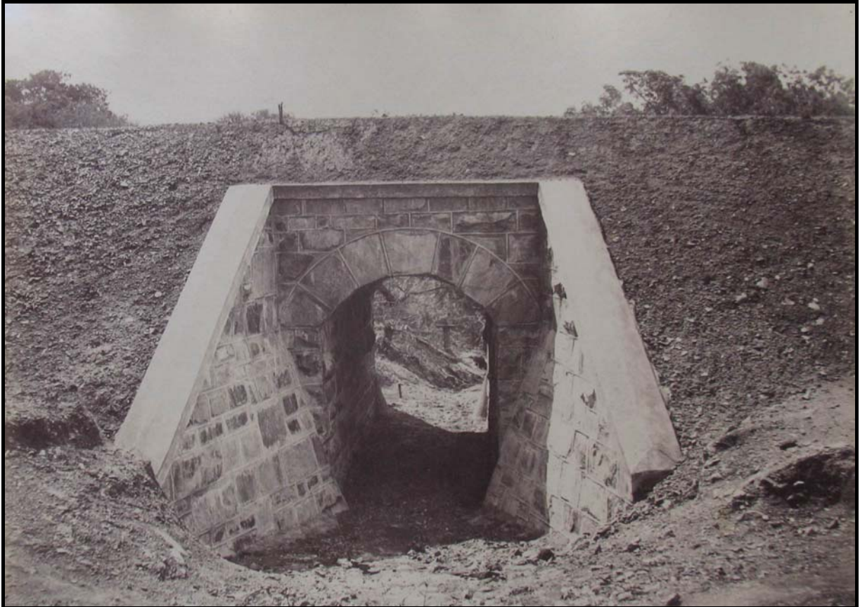
Fig. 6. One of the stone culverts shortly after completion (Photo: NCHM). Many such culverts still occur in the study area as part of the current railway line.
