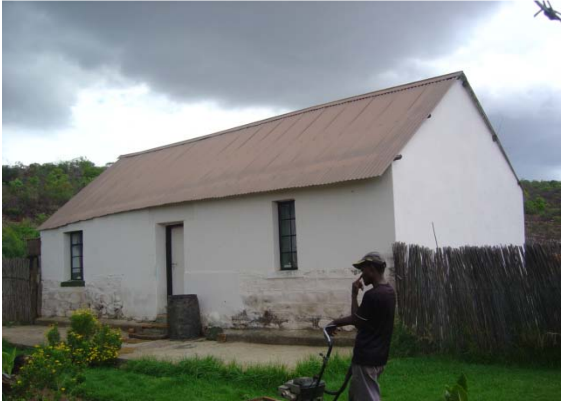
No. 3 Small original farmhouse
