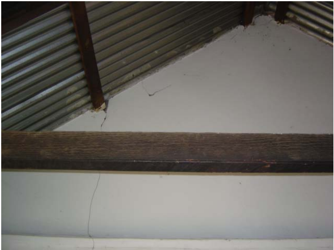
No.4 Hand cut beam
