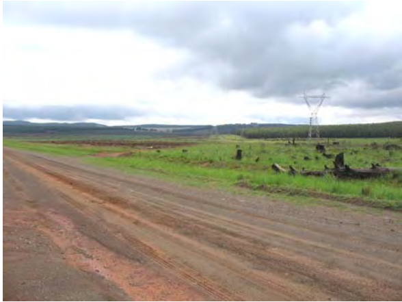
Fig 3. Route A along a power line and in the plantations of the farm Geluk 348 JT.
