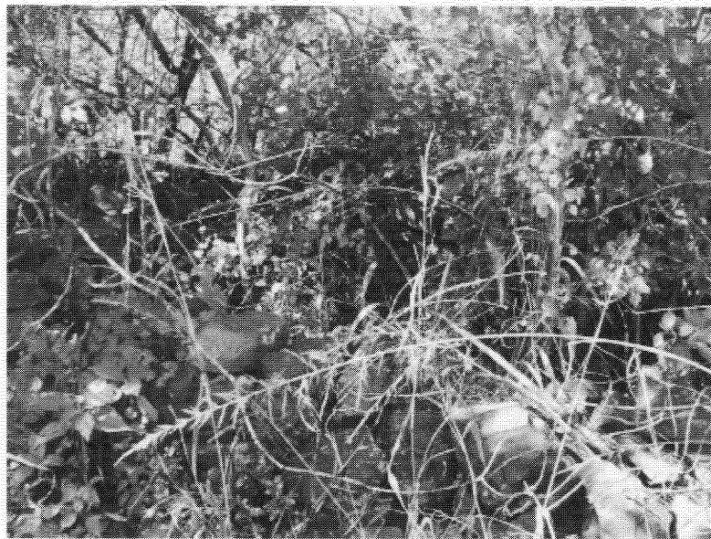
Fig 8. Site 4. Two collapsed circular stone walled structures.
