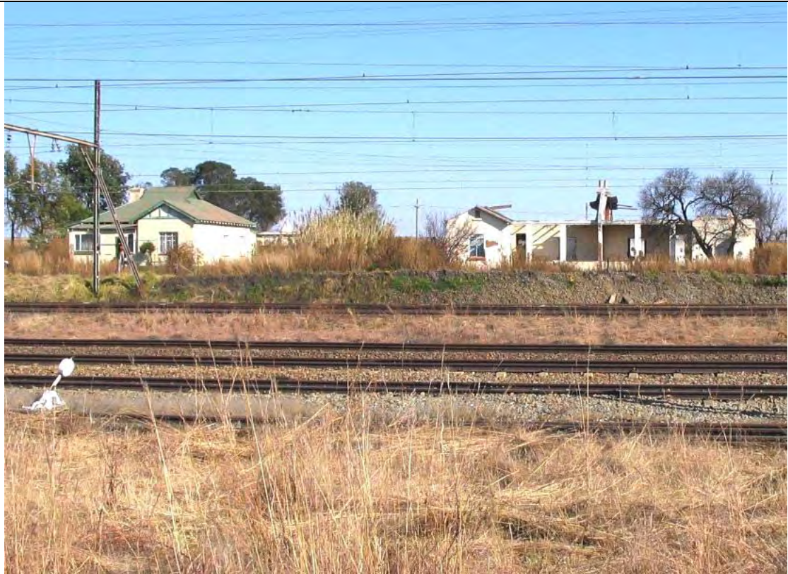
Fig 5. Heuvelfontein buildings opposite railway line.
