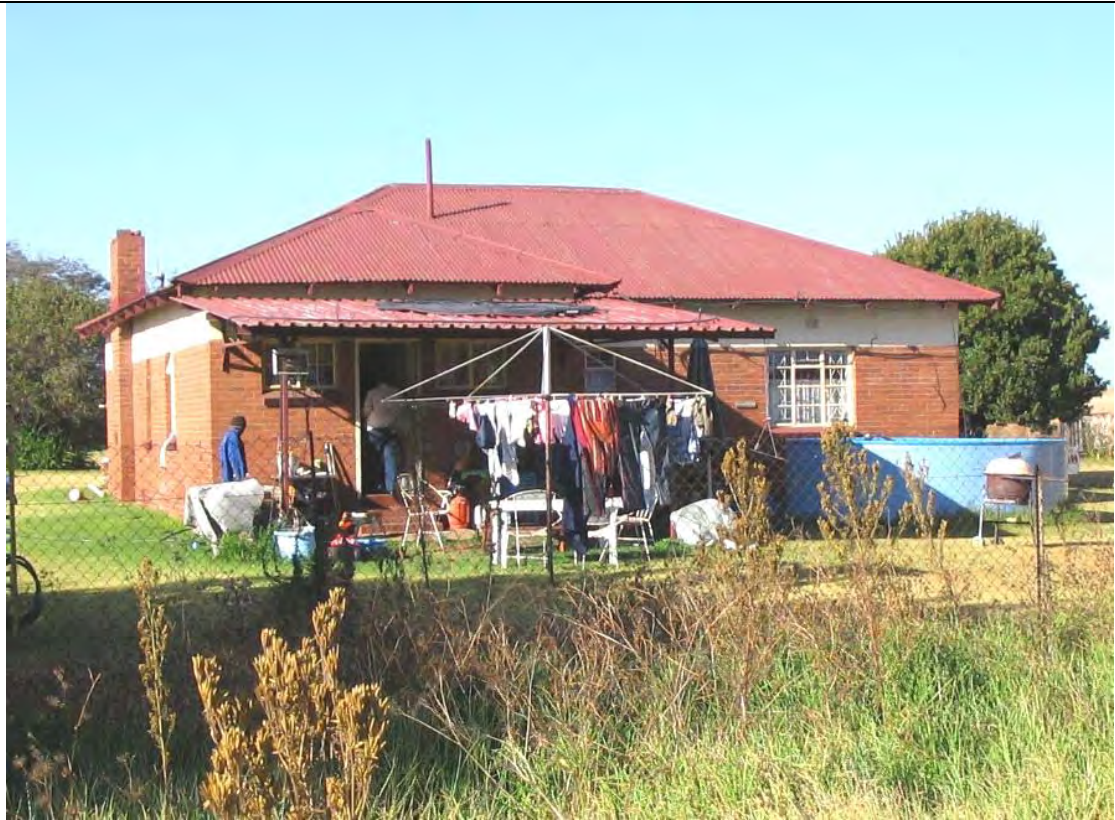
Fig 1. Mine house in original form – Vlakfontein / Klipfontein site.
