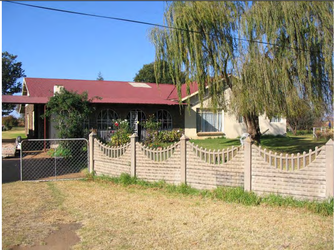
Fig 3. Altered Mine house – Vlakfontein / Klipfontein site.
