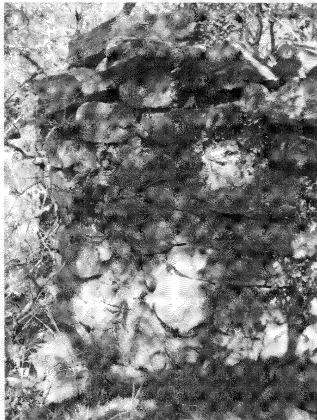
Fig. 19. Site 5. Mortar (mud) between wall stones.
