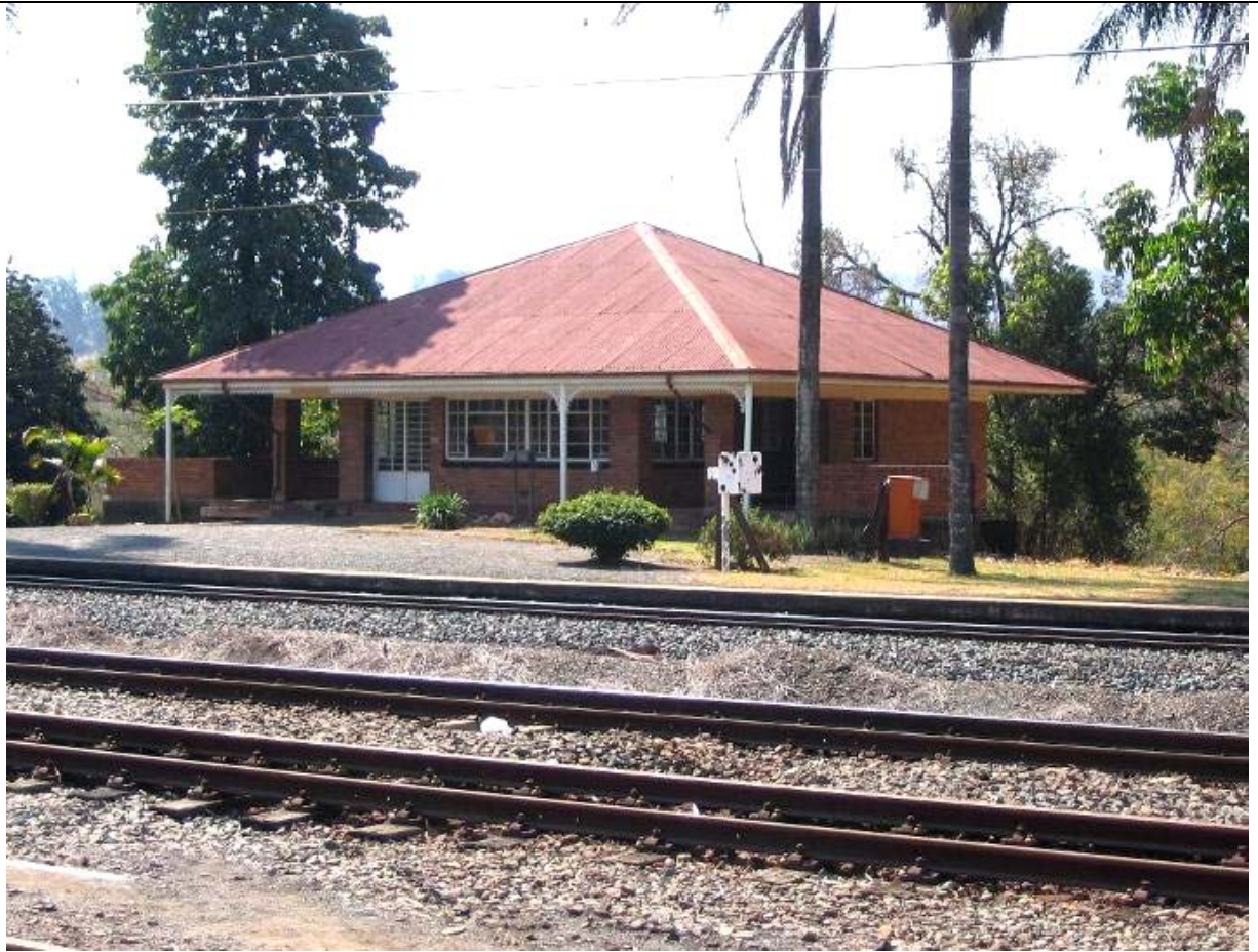
Fig 6. The Alkmaar Station building.
