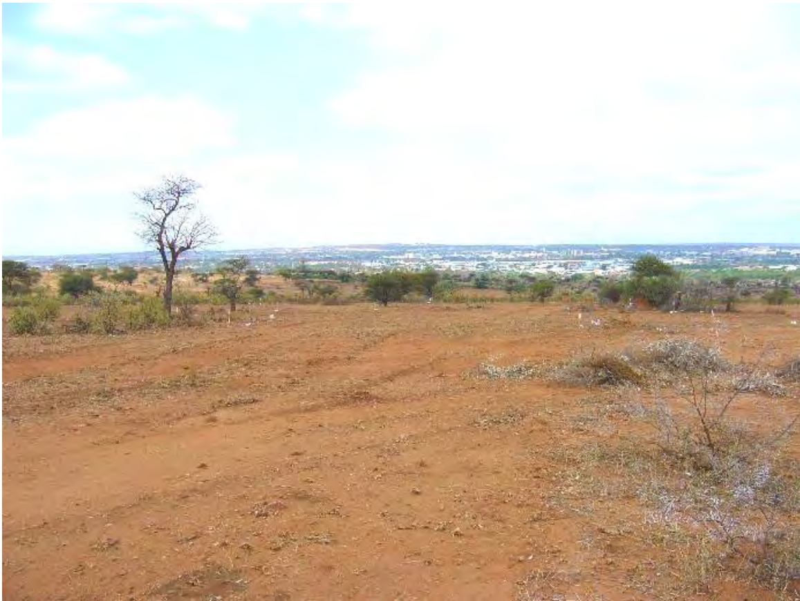
Fig 1. General view of the site – clearing of selected parts has commenced.
