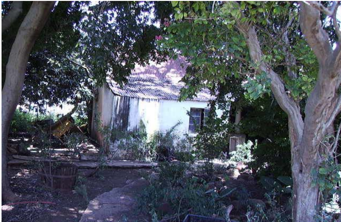
Figure 14. Eastern wing of the 1910's house.
