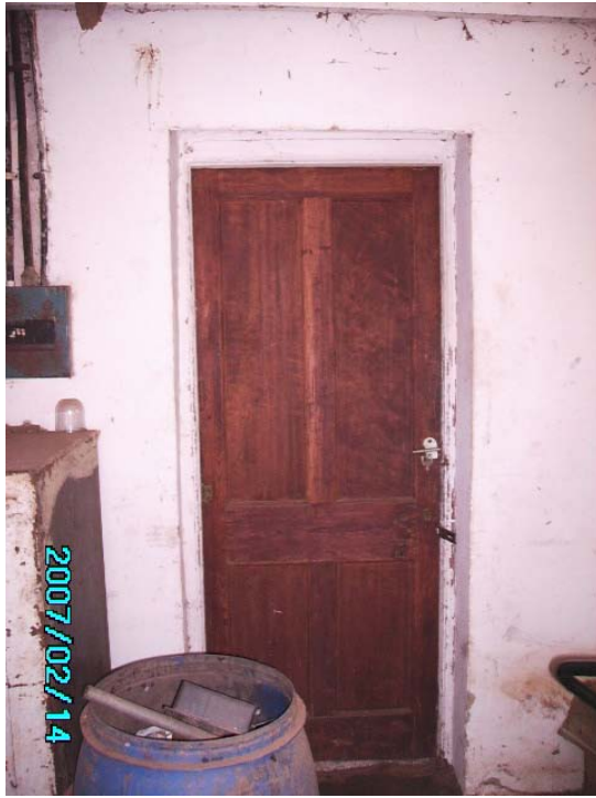
Figure 05. The general preservation of architectural detail is rather poor. Doors, locks frames and windows were originally of poor quality and much of the originals were replaced or are damaged beyond repair
