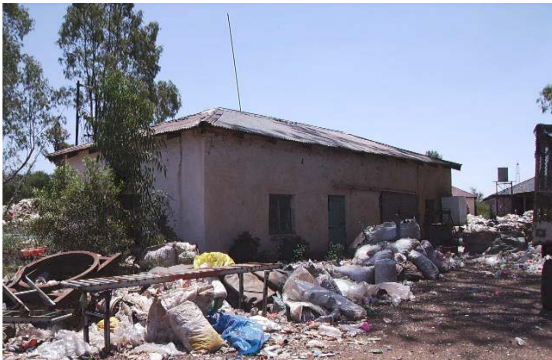
Figure 04. The 1930's house. This structure is also in a bad state of repair.
