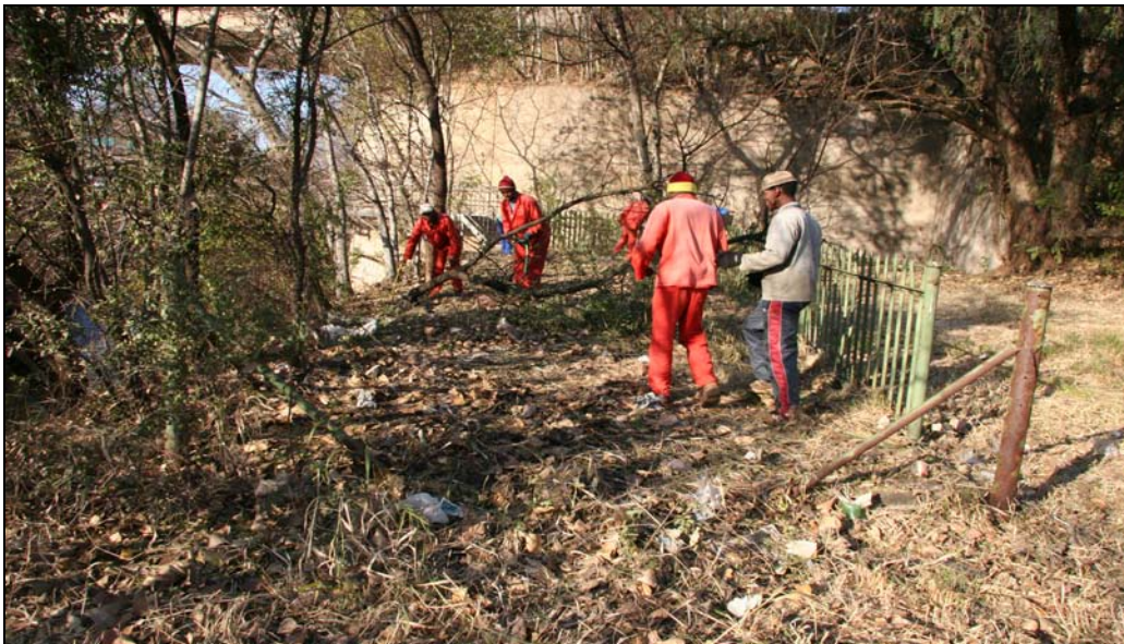
Figure 1: General view of site and clearing in progress
