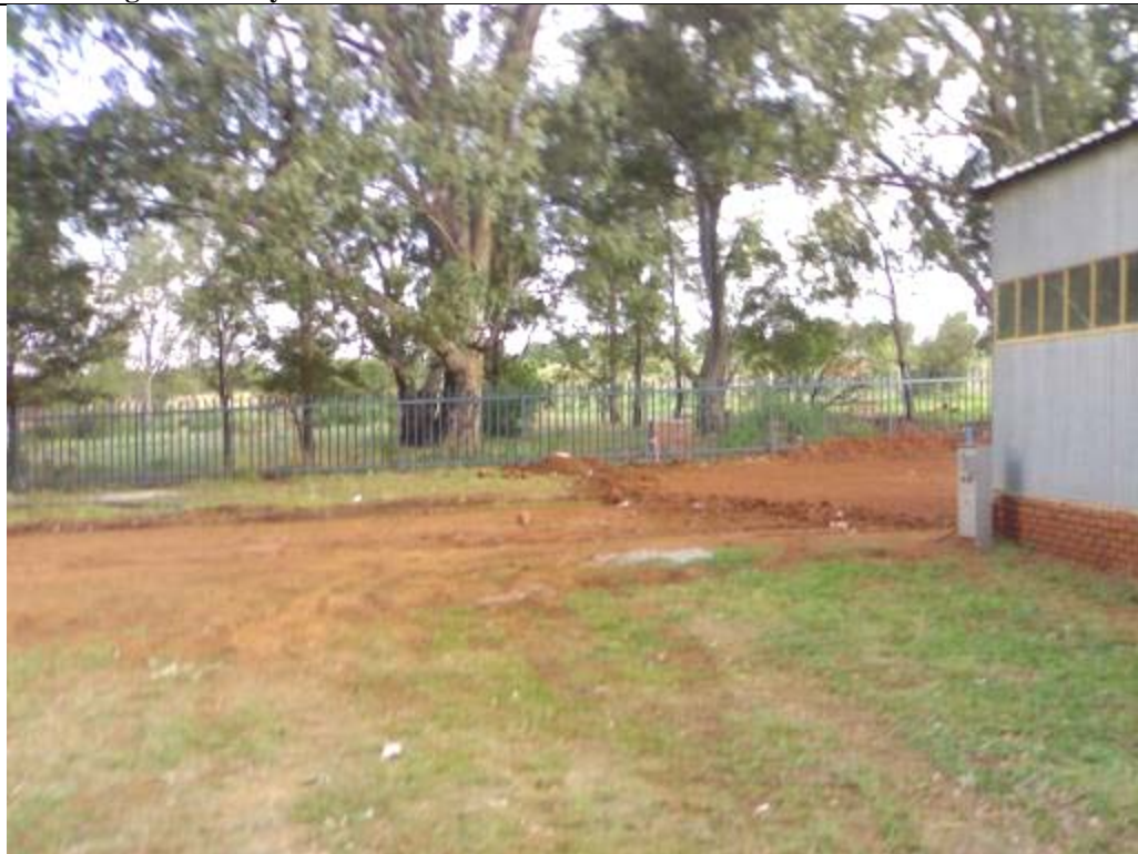
Figure 7: Cleared area for the construction of the reservoir
