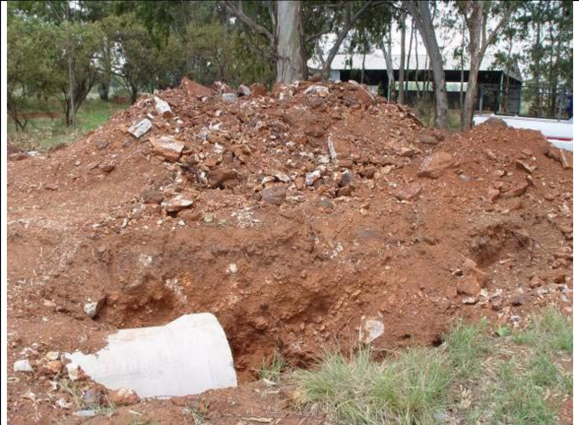
Figure 4: Large hole for storm water drainage
