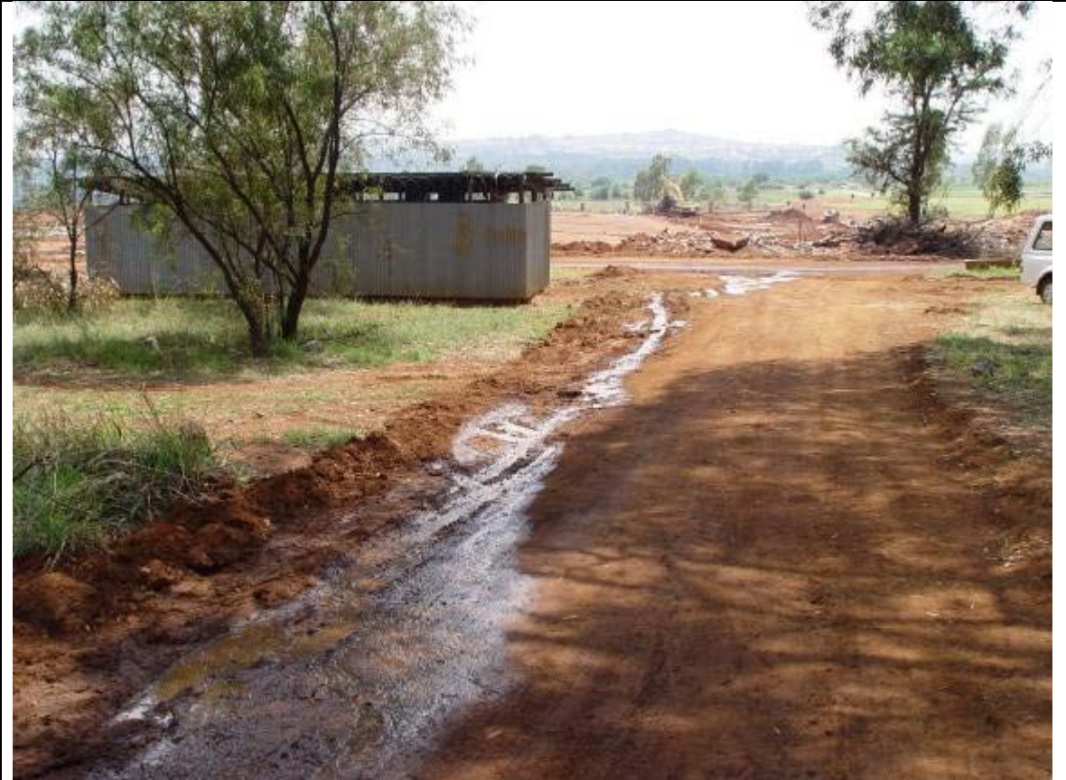
Figure 3: Access road to the borehole and tap
