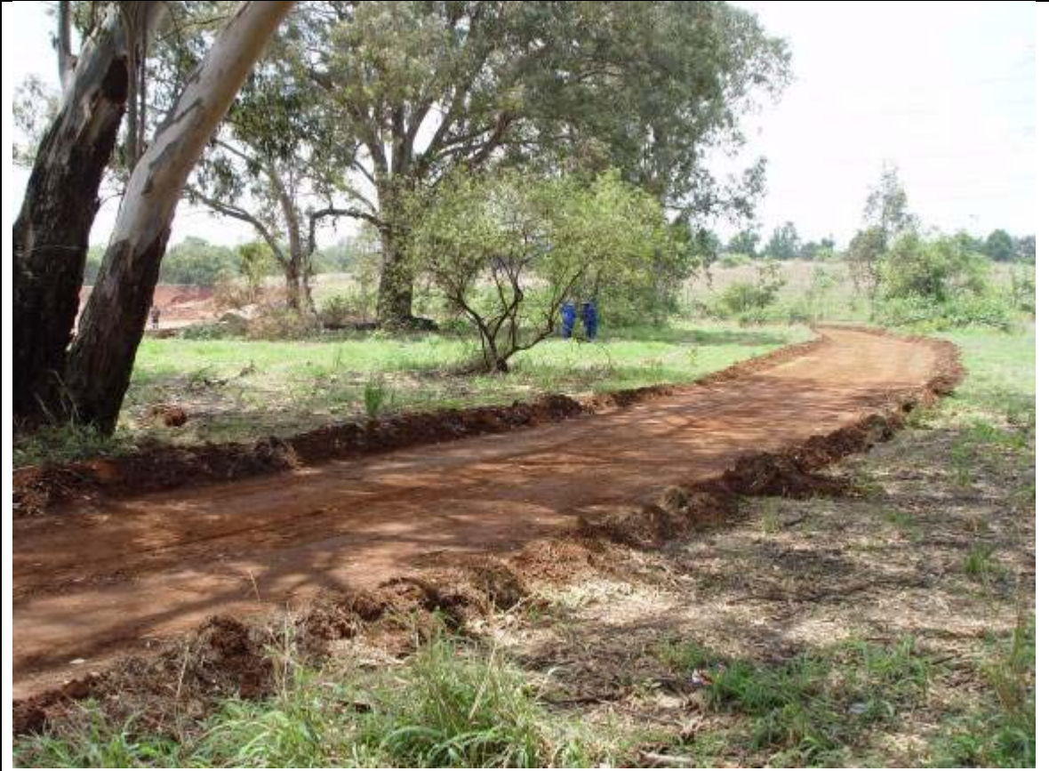
Figure 5: New access road
