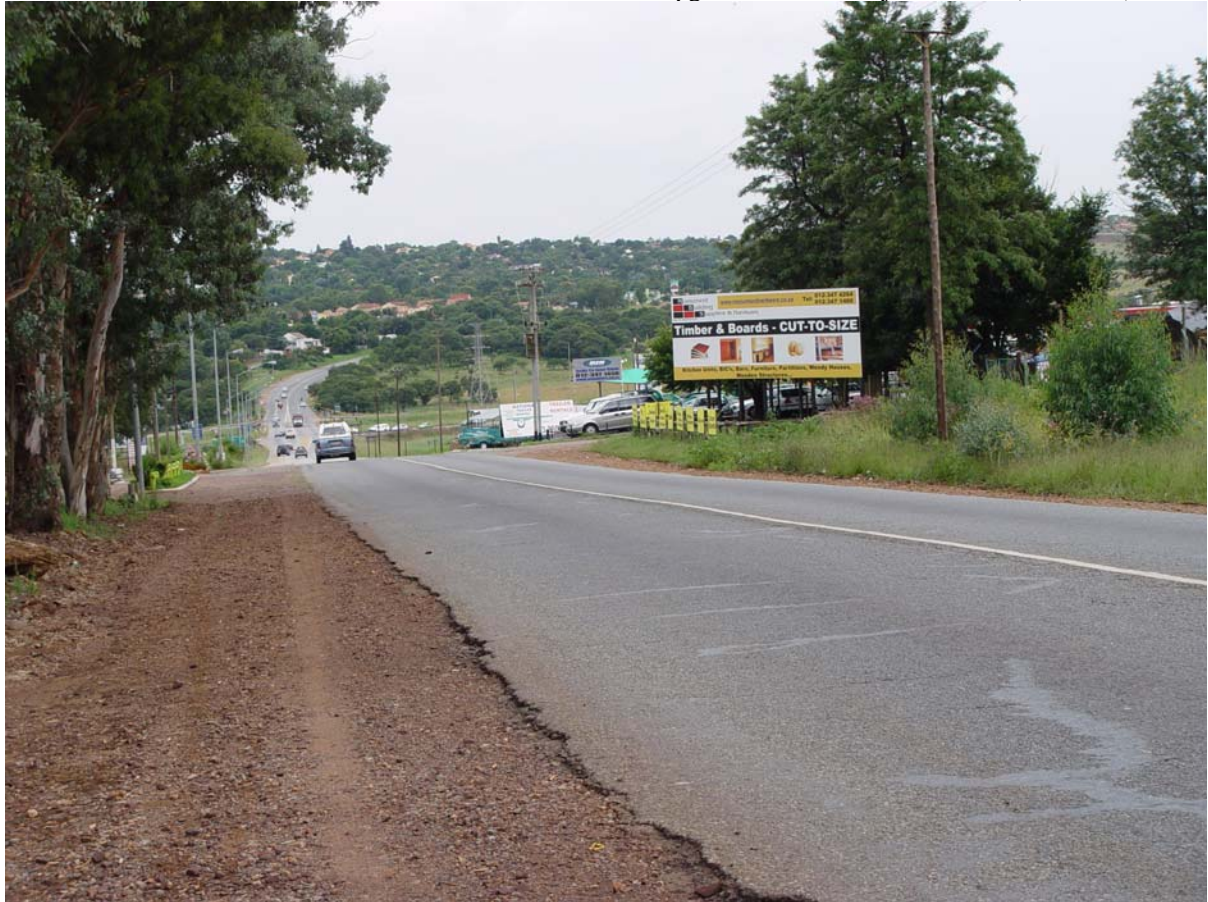
Figure 2: State of the road reserve: Hans Strijdom Road
