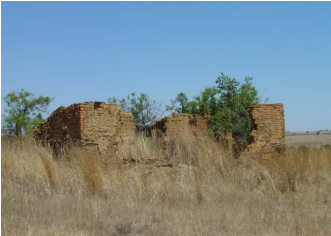
No. 2 Remains of one of the oldest farm workers houses
