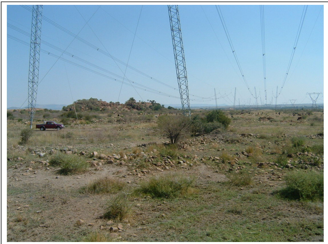
Figure 3- Site LIA01 underneath Eskom's existing power lines. Site LIA01 was damaged when these power lines were constructed in the past (above)..
