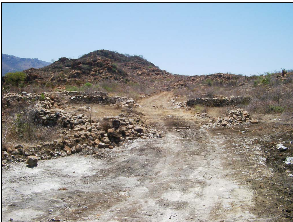
Figure 3. Damaged to one of the stone walled sites. This is not the only such occurrence.
