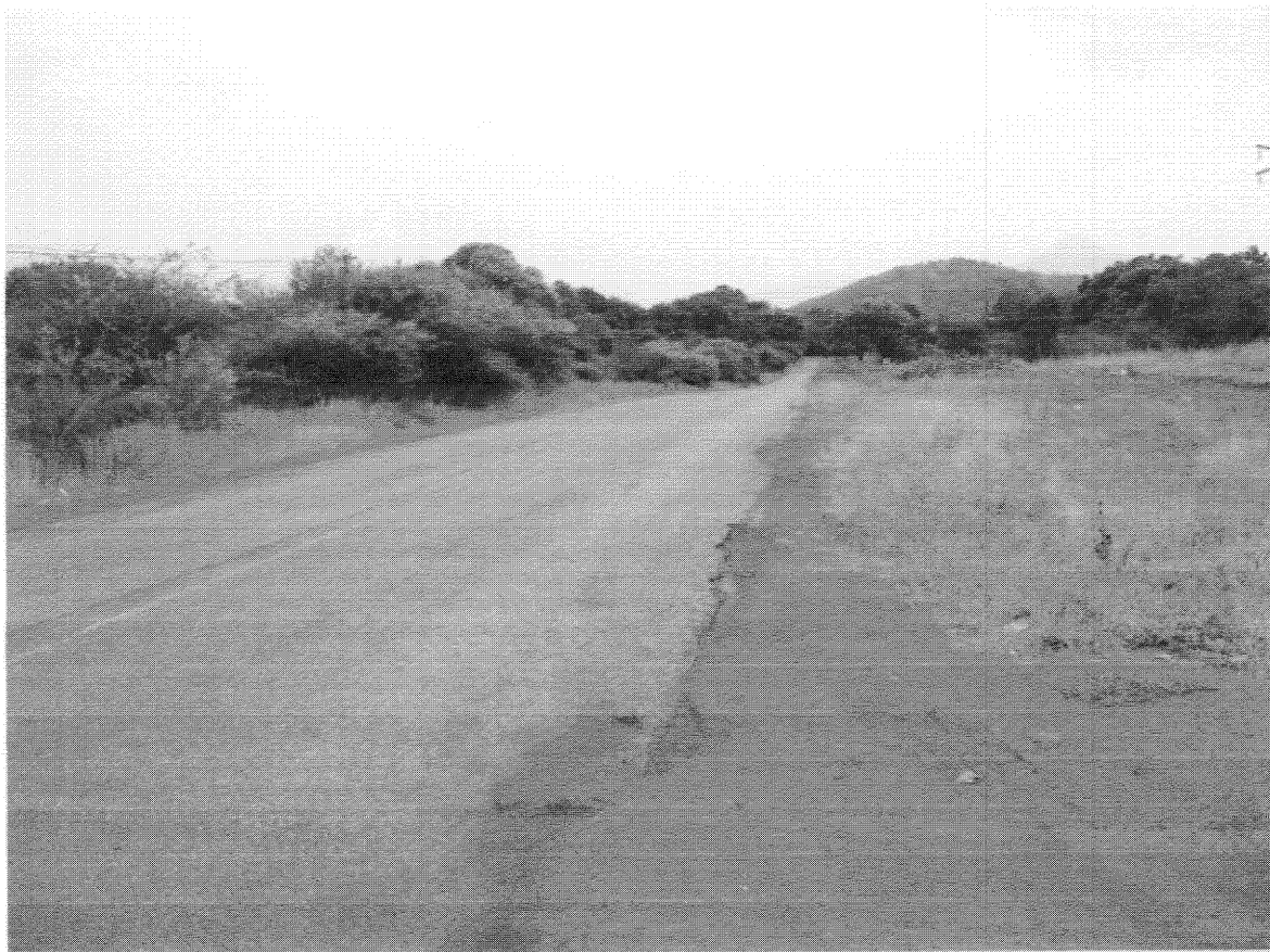
Photo 8: Road upgrade end.
