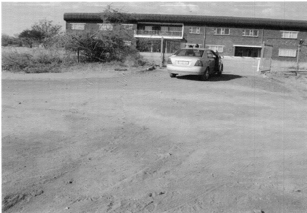
Figure 3: View of the Sekhukhune College of education main gate where the proposed road ends.
