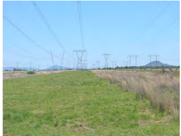
Fig 2. Existing power lines.
