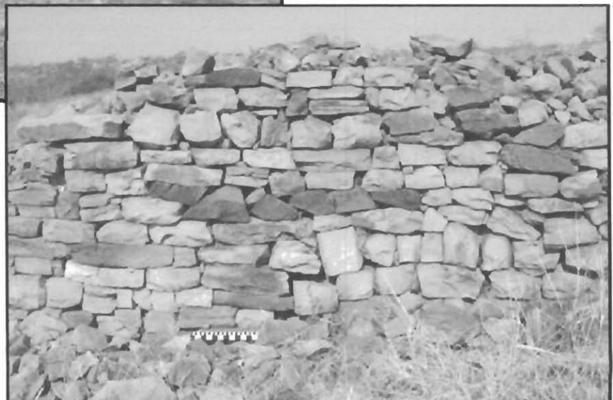
Photo 12. Stone Wall 1 on site Map 21.
