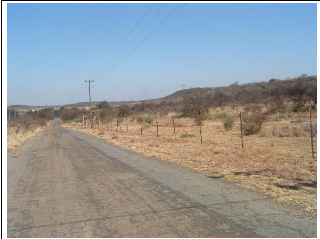
Figure 1- The low range of hills referred to as 'Houtkop' in the Project Area will be crossed by both the water as well as the sewage pipe line corridors. This view is from the Rand Water's reservoirs in the north towards the south (above).
