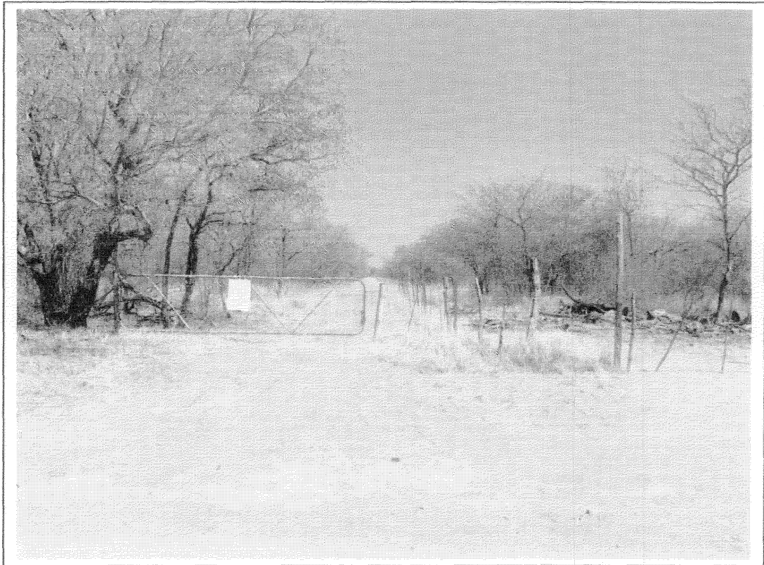
Figure 5- The last stretch of the proposed new power line running between the Matlabas and the Bulge Substations. Stretch EF is visible in the background where the proposed new Bulge Substation will be located (above).
