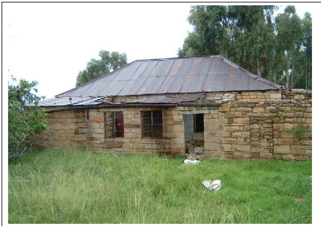
Figure 6- The farmstead in Site SCH01 consists of a rectangular core structure build with sandstone. Note the extensions (lean-to's) constructed on at least two sides of the house. This is the 'normal way' through which the core of the farmstead was extended over time. This farmstead is associated with a shed and with a graveyard.
