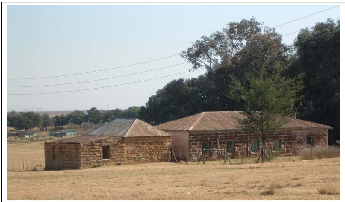
Figure 13- A sandstone and a ferricrete house next to each other (above). Note the lean-to constructed against the square structure. The entire ferricrete house was built with dressed ferricrete, which was shaped in a standard size so that it could be laid in level layers. The mortar between the layers was whitewashed. The two houses are also associated with a historical graveyard.
