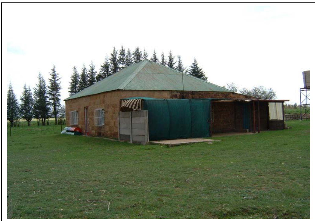
Figure 9- The farmstead in Site SCH02 was built with sandstone while the lean-to was also constructed with ferricrete.
