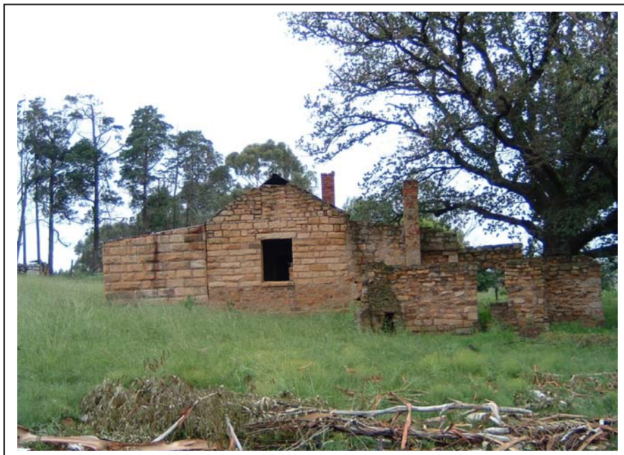
Figure 12- The excellently preserved remains of a sandstone farmstead associated with Site SCH04. Note the large (historical) Oak tree next to the house. The house has been extended several times from its original core, mainly by means of lean-to's (above).
