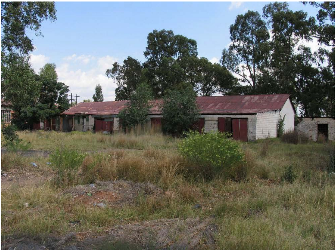
Fig. 5. Part of the workshop/wagon sheds.
