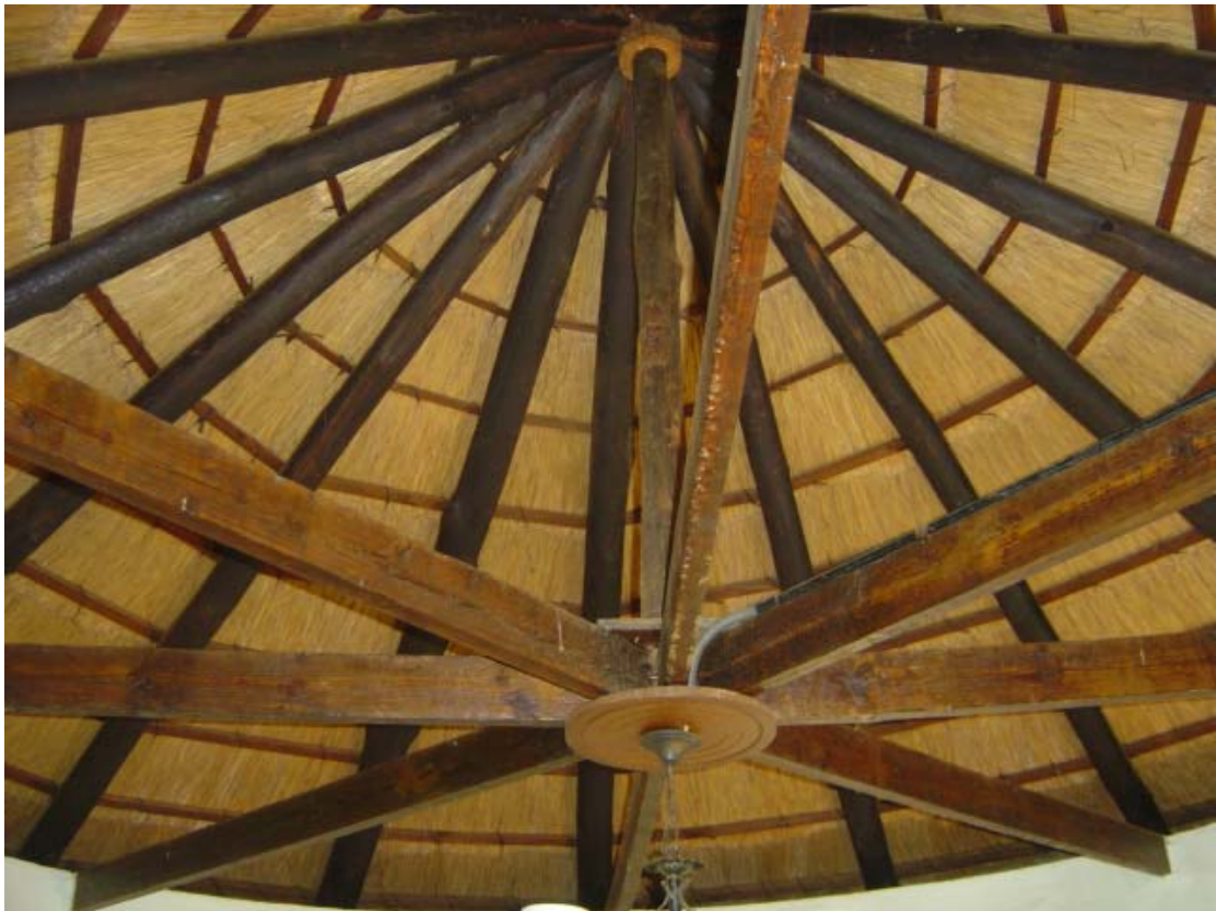
Detail of the wooden roof construction
