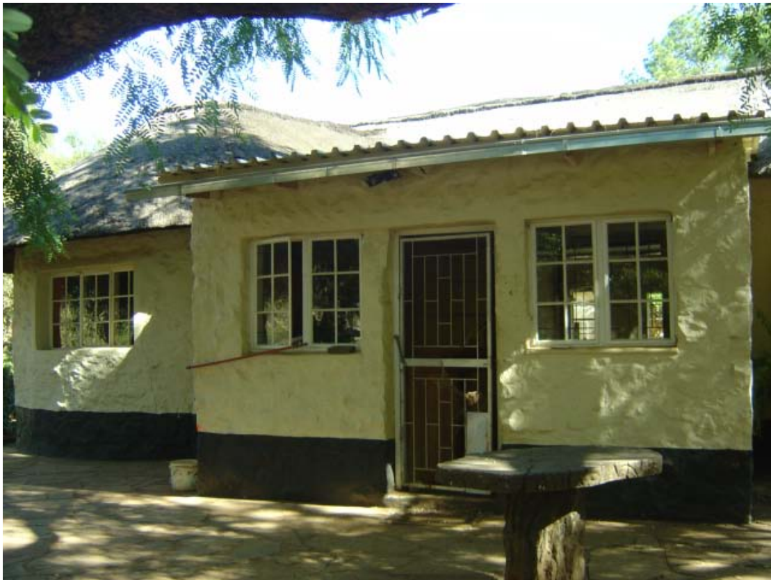
The new kitchen added on the eastern side
