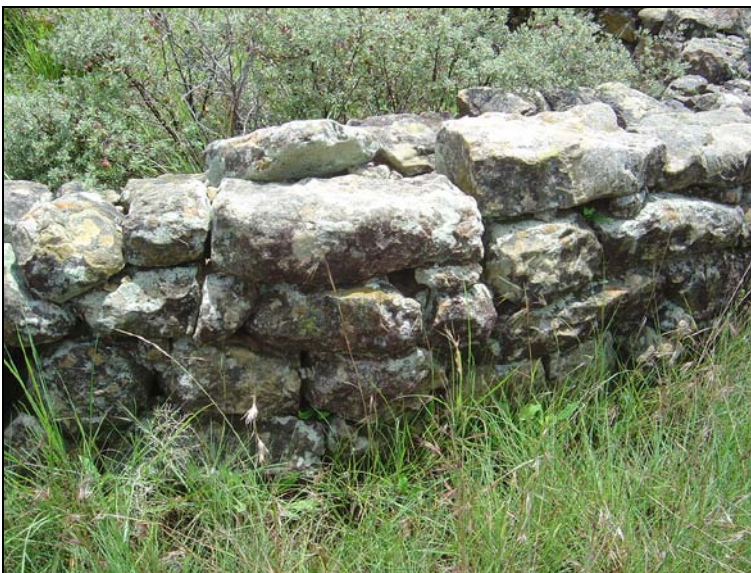
Fig.6 The stone wall of one of the structures.
