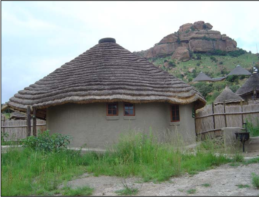
Fig. 3 View from down below facing up the slope towards the present office building and parking area. Korfskop at the back.
