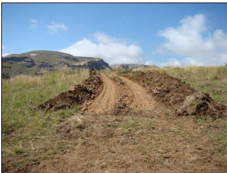
Fig.2 Point A site of the bio-filter plant.
