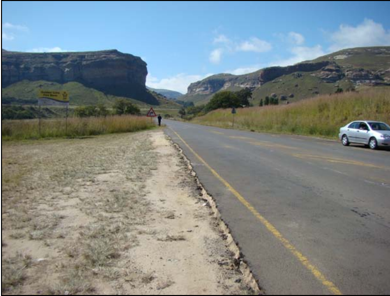
Fig.5 Facing east from the Entrance Gate at Point B.
