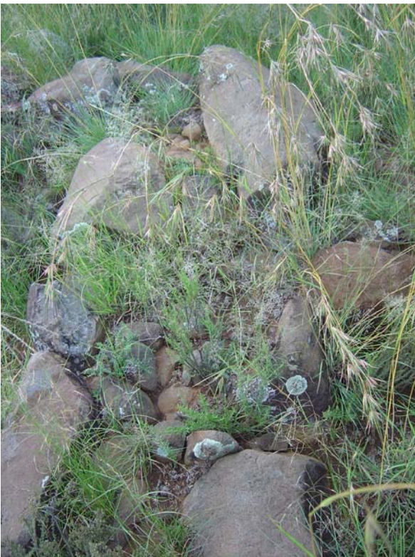
Fig.2 Wall is constructed with 2 sides and a centre fill of small stones.
