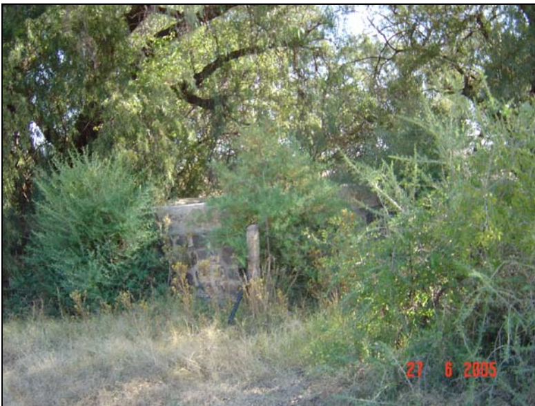
Fig.14 Stone-walled water reservoir at entrance gate.
